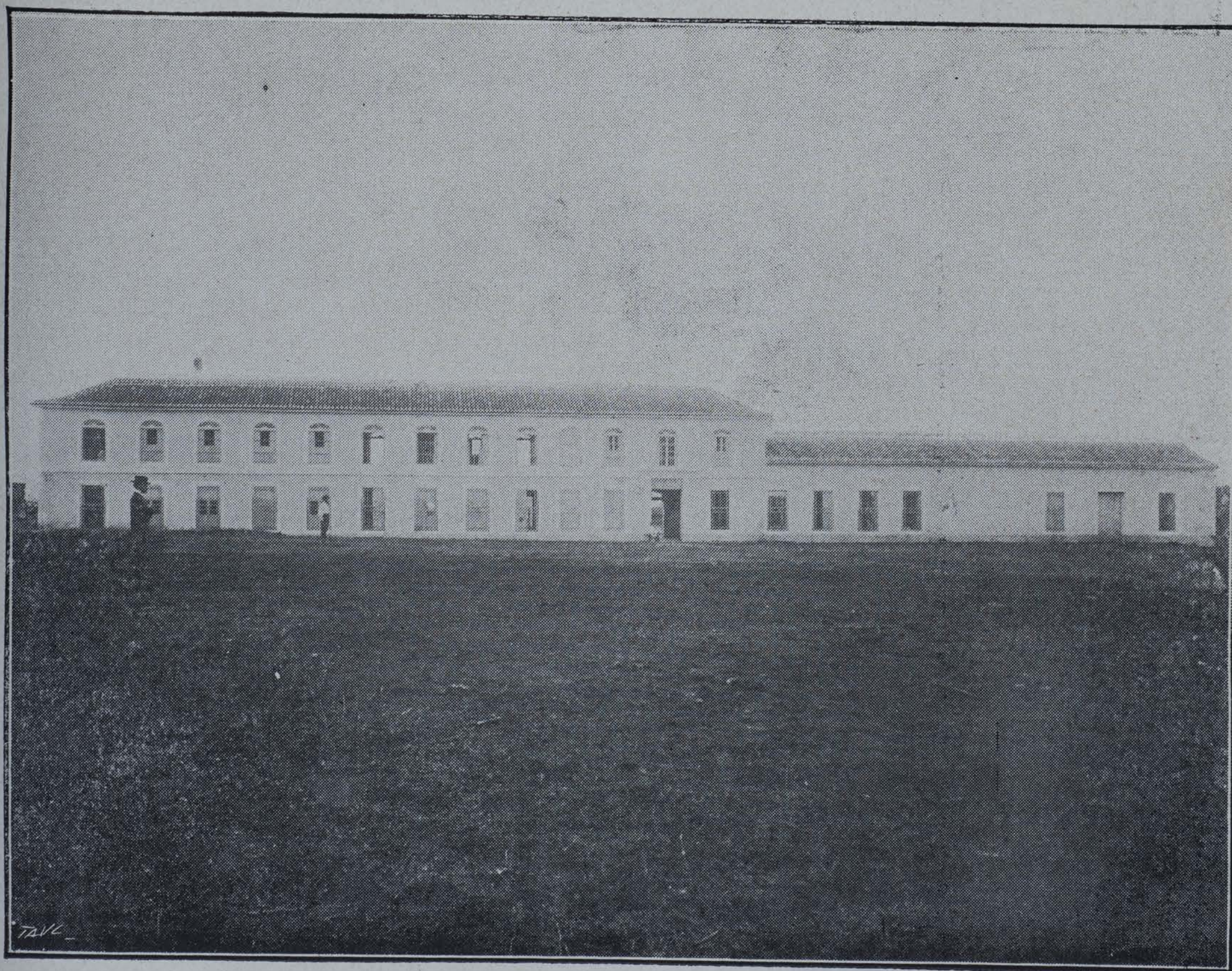
FACHADA DEL HOSPITAL CIVIL "GENERAL WOOD", TRINIDAD
